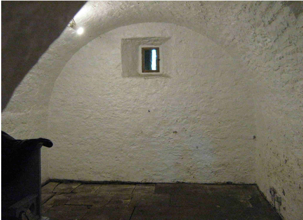
Plate 1. Interior of the vaulted basement of the Pele looking west, showing a loop hole. The Test Pit was excavated in the left-hand (south-west) corner.
