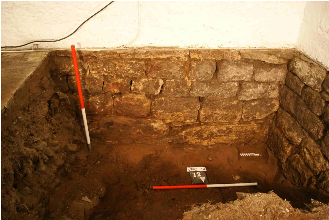
Plate 7. Inner face of the south wall of the Pele, showing base course and small underlying stones in truncated construction cut. Scales 1m.
