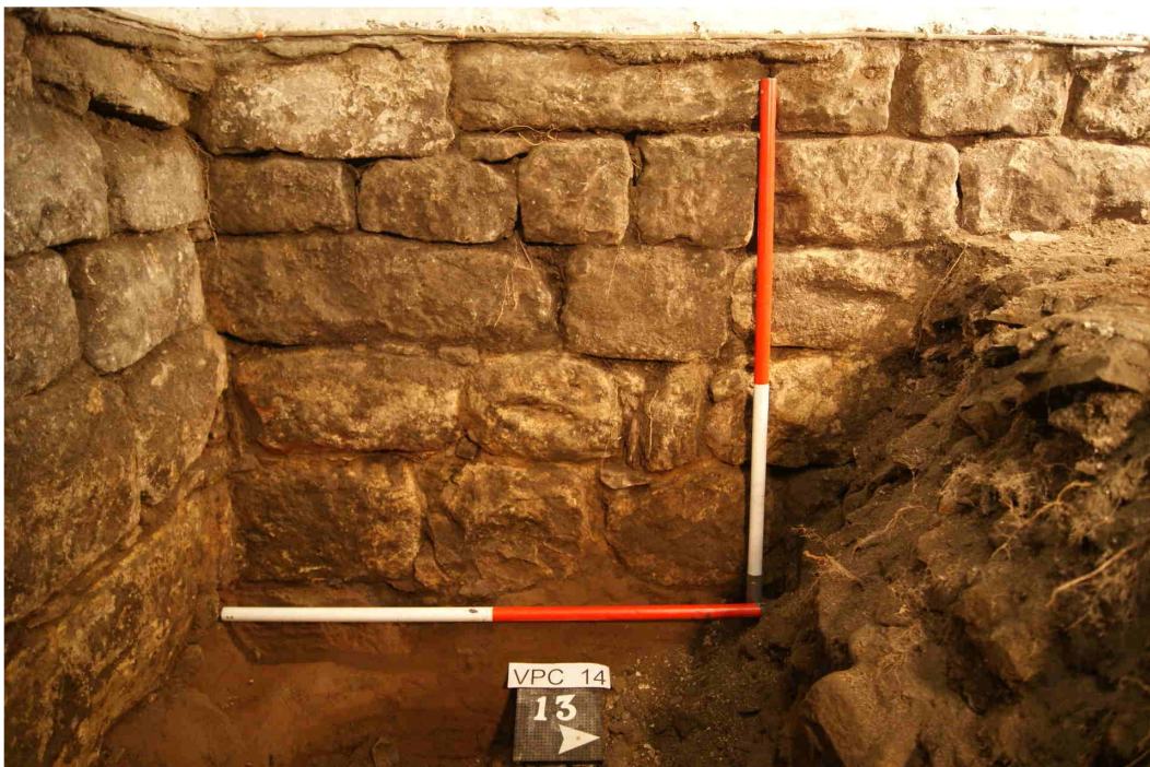
Plate 8. Inner face of west wall of the Pele <13> and junction with south wall <12>, showing base course resting on natural alluvial sandy clay and possible construction joint (see Figure 14). Scales 1m.
