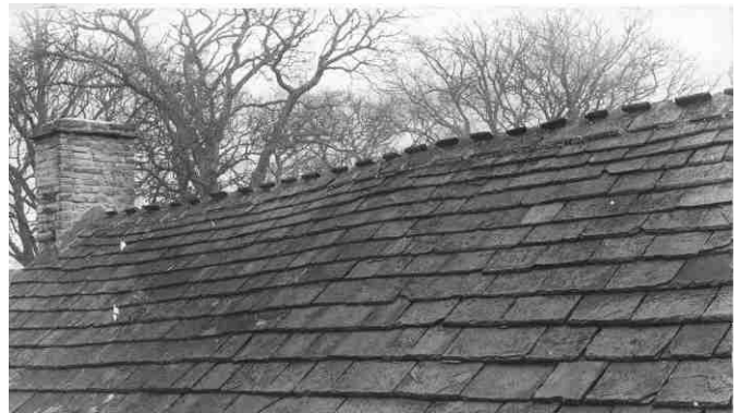
Figure 7. Left: a 'wrestler' tile from context <6> showing the notches where the tiles interlocked. Above: 'wrestlers' in situ forming a roof-ridge, with stone flags of graduated sizes.
